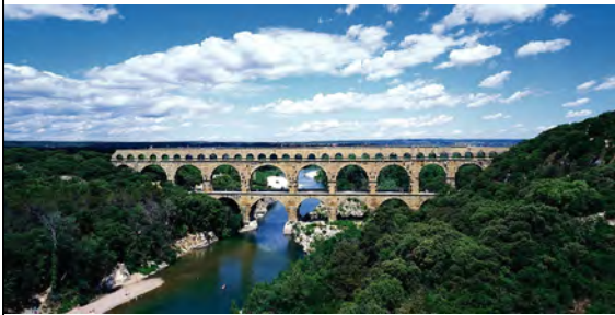
Figure 10-33 Pont-du-Gard, Nîmes, France, ca. 16 BCE.
